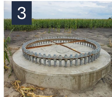
3 Foundation installation
