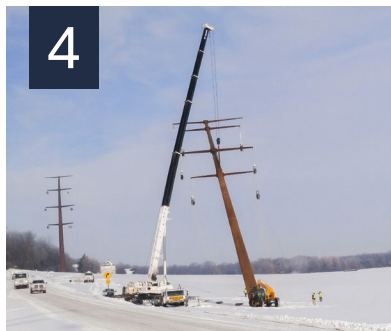
4 Assemble and set structures
