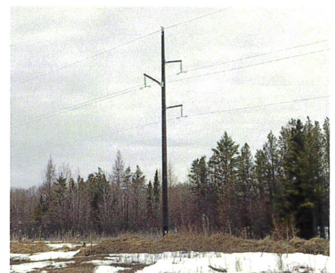
Example of proposed 69-kV line structure
